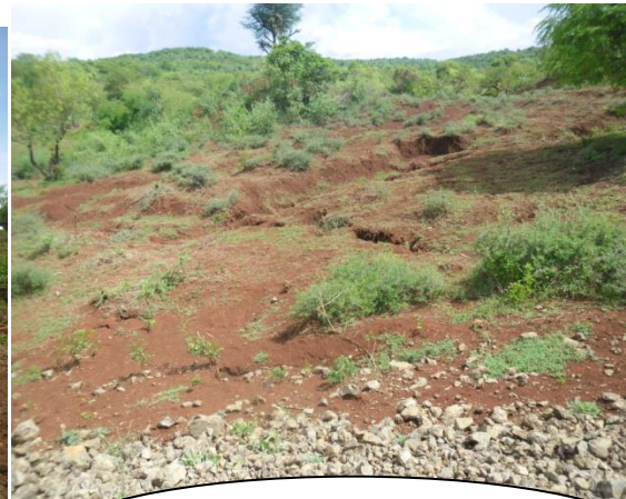
Erosion Problem at Malka Amana Kebele
