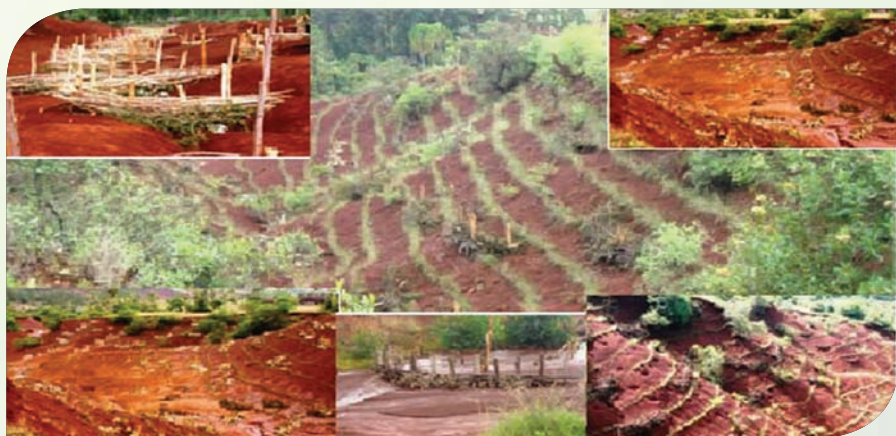
Combination of check dam and grass strip planting on a highly degraded hill
