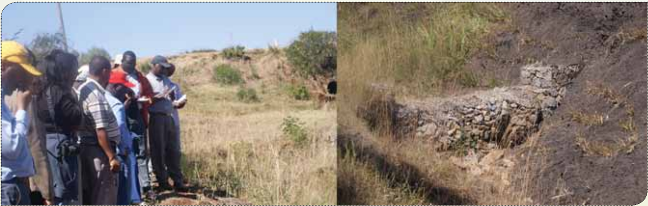
Parliamentarians, zonal and woreda officials visiting Gilgel Gibe Dam I and SLUF's project Site-treatment of gully erosion.
